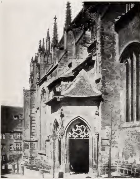
Illus. 287.—Rothenburg. Standpoint XI on Fold Plan III. St. Jacob's Church; example of Gothic building.
